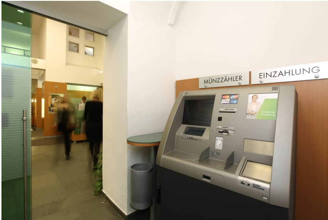
KePlus X6se at the Lofer branch of the Raiffeisen bank
