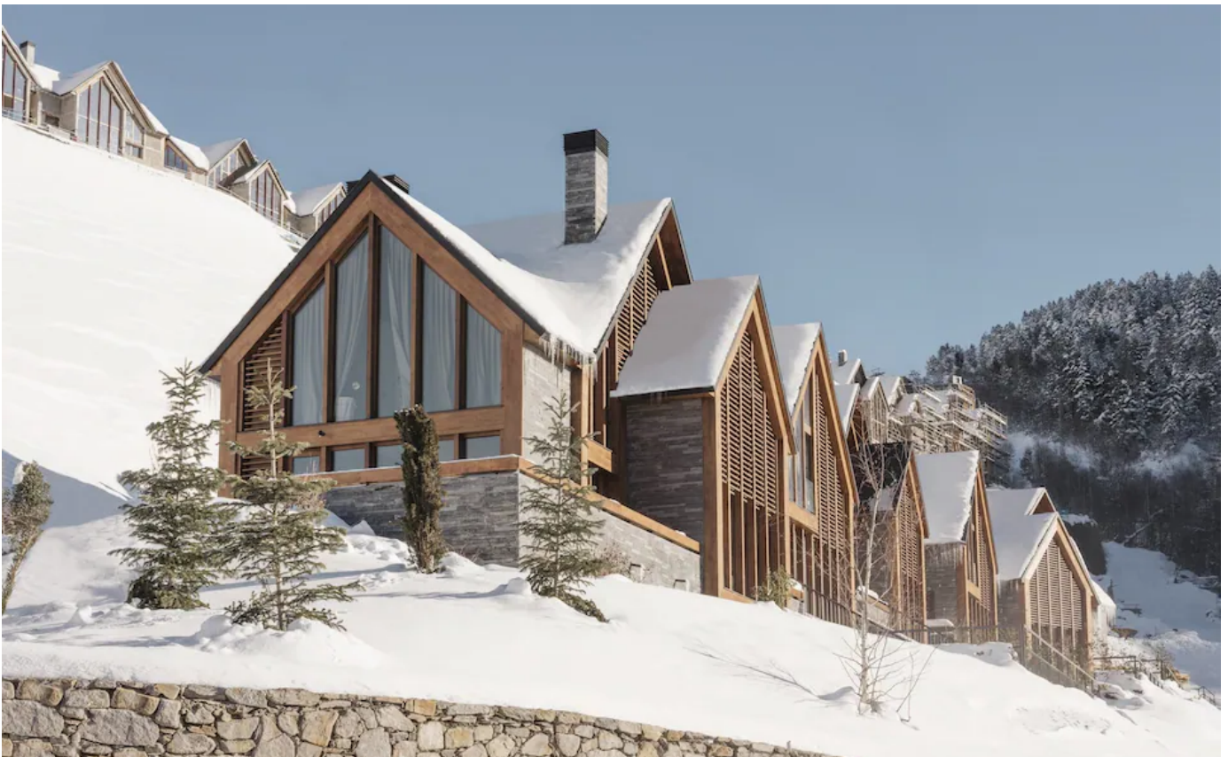
Chalet Timok is part of a new development of high-end residences in the Pleta Arriù area
