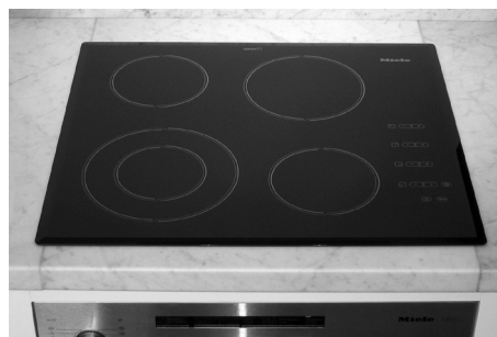
Split cut-out for a hob installed in a stone worktop. Note the joints between the front and rear strips and the surrounding worktops. All worktops must be sealed at the rear and sides to prevent moisture ingress.
