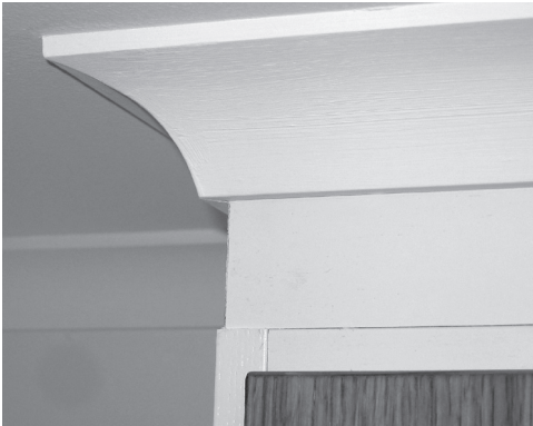
Ceiling connection panel installed between the wall unit and the moulding. Note that the ceiling connection panel is recessed a few millimetres in relation to the wall unit.
