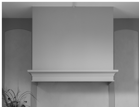
The upper section of the Sundby extractor hood is to be filled and painted on site.
