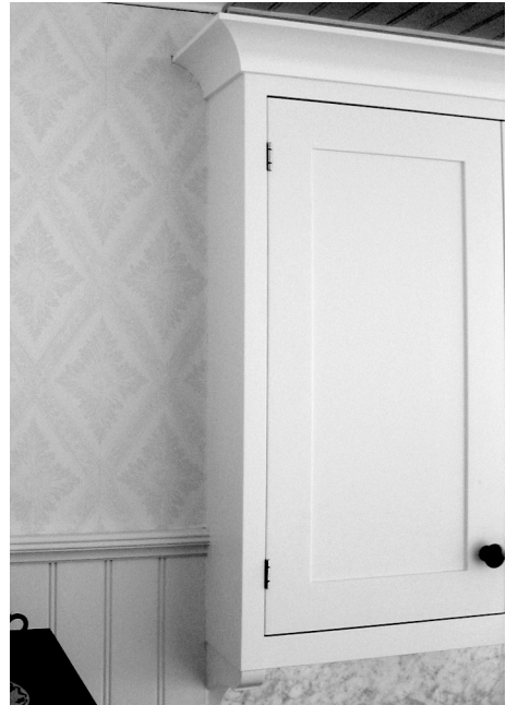
Covering side mounted to the side of a wall unit.
