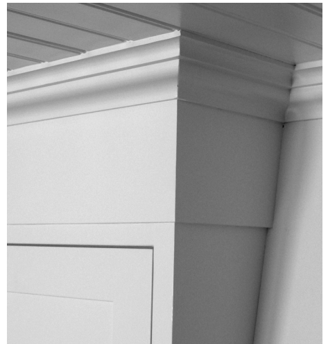
Filler panel between ceiling batten and the upper part of a wall unit.
