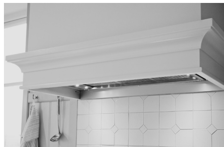
The Sundby fan hood, the upper part of the hood is spackled and painted on site.
