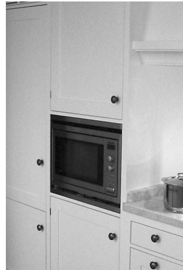
Tall unit for integrated oven or micro. Note the front of the micro is flush with the front edges of the frame.
