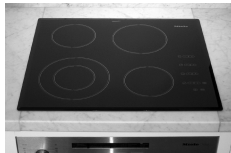
Split cutout for hob in a stone worktop. Note the joints between the front and rear sections and surrounding top.
