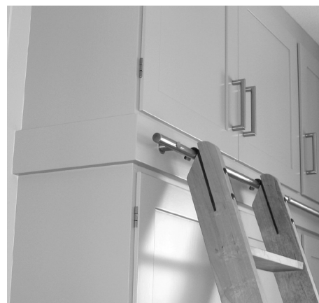
Ladder leaning on a rail. Note that the rail is fixed to the spacer batten between the units.
