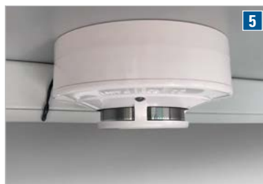
Smoke detector and temperature sensor.
