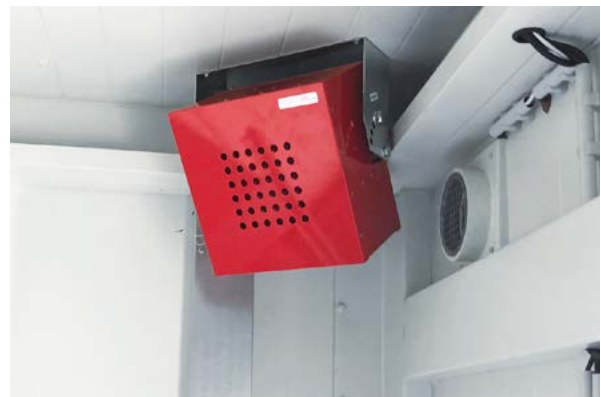
The aerosol extinguishing system is triggered by temperature and effectively interrupts the chemical combustion process within 4.5 - 15 seconds, depending on model.
