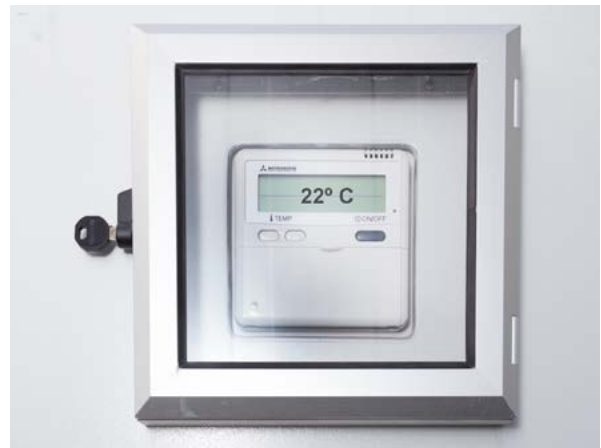
Temperature display for an air-conditioned hazardous materials store.
