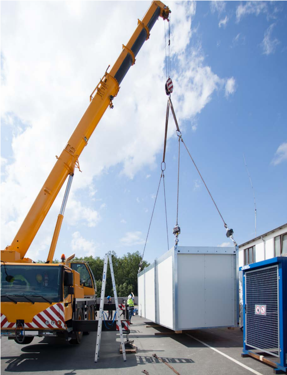
A crane is usually used to install a hazardous materials store outdoors.
