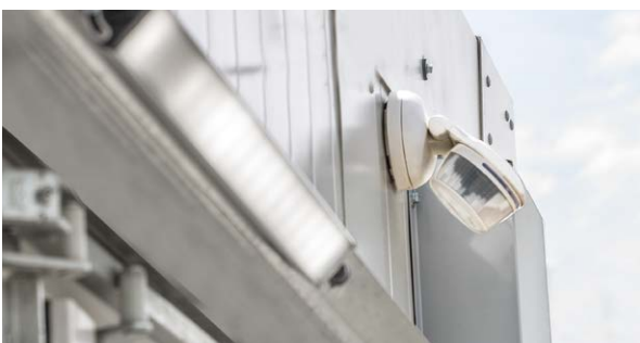
External lighting with motion sensor.
