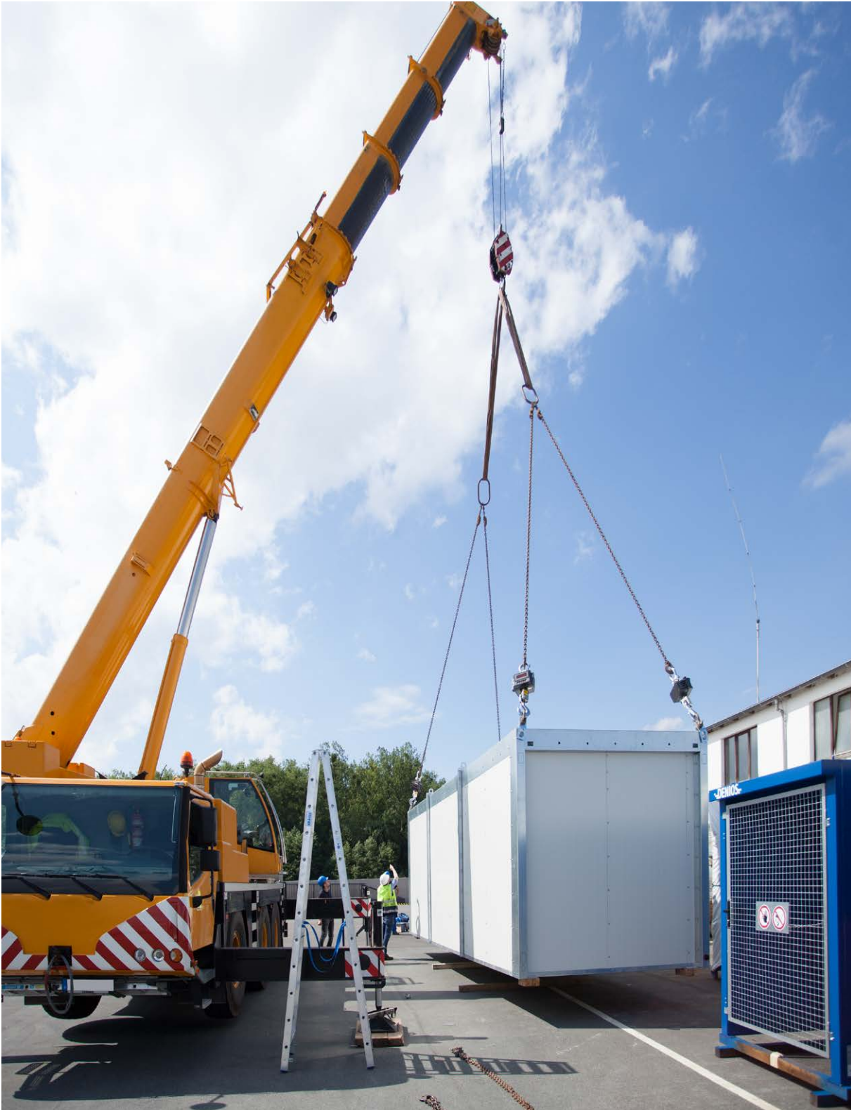
A crane is usually used to install a heat chamber outdoors.
