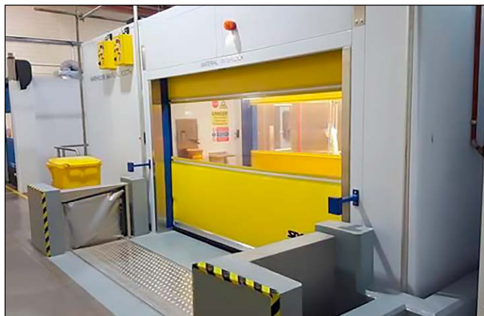
All these barriers are FM Approved for flammable liquid retention.
