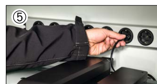
Power strip with metal housing and earthed sockets
