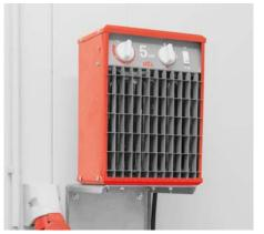
In combination with the thermal insulation, the 5 kW heating system ensures an indoor temperature of +5 °C at -15 °C outside.
