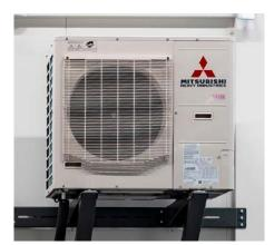
In the standard version, the air conditioning system achieves indoor temperatures of +15 °C at an outdoor temperature of up to -15 °C and +20 °C at an outdoor temperature of up to +35 °C.
