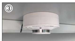
Smoke detector and temperature sensor
