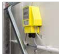
Air extraction monitoring for air exchange > 2.0/h
