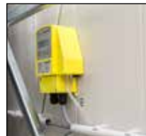
Air extraction monitoring for air exchange > 2.0/h
