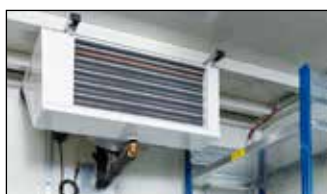
Climate control equipment for precision tempering in the inner room
