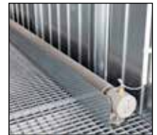
Finned tube heater with impact protection
