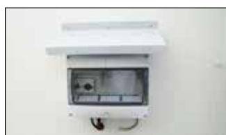
Sub-distribution unit (e.g. when sockets are used)
