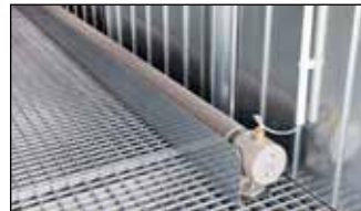
Finned tube heater with impact protection
