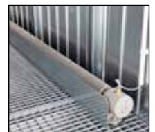
Finned tube heater with impact protection
