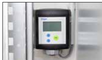
System monitoring / gas warning detector
