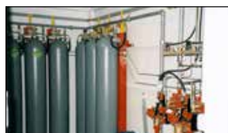
CO 2 extinguishing equipment
