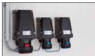
Sockets for connection of additional works equipment (230 V or 400 V, 50 Hz.)
