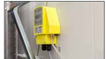
Air extraction monitoring for air exchange > 2.0/h
