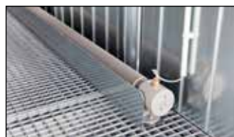
Finned tube heater with integral safety temperature limiter and impact protection panel
