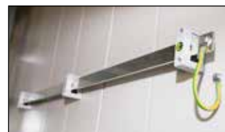
Earthing rails inside the technical room system
