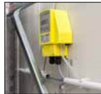
Air extraction monitoring for air exchange > 2.0/h
