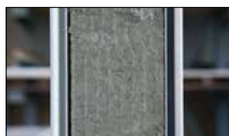
Fire protection panels in non-combustible A class material (mineral wool panels)
