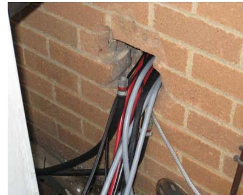
*ECU control cables entering the testcell through the wall*
