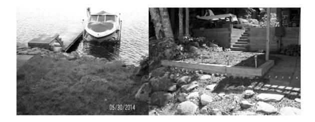
The next pair of photos shows the north side of our home with little ground cover and the outlet of a buried storm drain. We built a three-tiered retaining wall to slow rain water running off the roof (we intentionally leave all the leaf debris above the wall). We backfilled the area above the ties with a clean rock and covered them with landscape fabric. By leveling the area, we distribute the roof runoff more evenly, while landscape fabric and cleaned rocks filter the drain pipe outflow.
