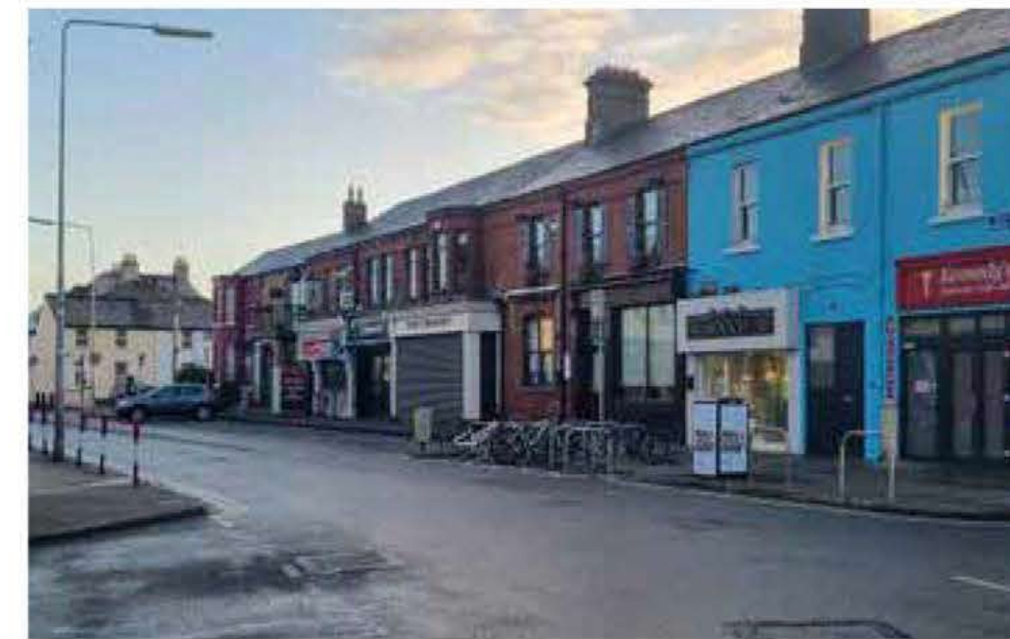
Vernon Avenue - existing
