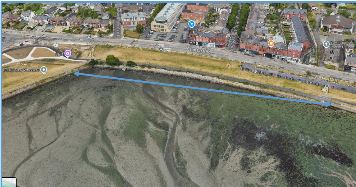
Above: the 300 metres section of coastline (adjacent to the Clontarf Road) which his currently protected to a degree by the in-situ sandbags.
