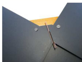
Nailing in the batten and placing of the hook in the joint in-between 2 slates
