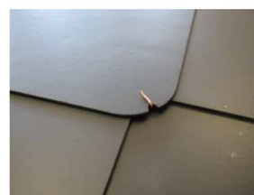
Placing of the next slate on the hook
