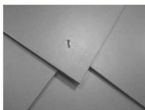
Placing of the next slate over the disc rivet and bending of the disc rivet, not too strong so that movement of the slate is still possible
