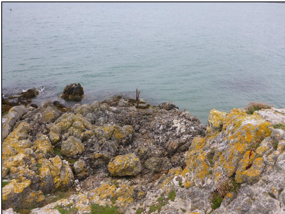
Plate 9 Iron railing at western landing place
