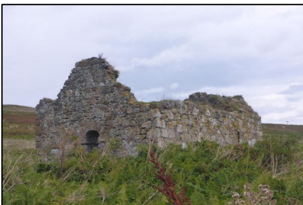
Plate 31 West gable and south wall of nave, St Nessian's Church
