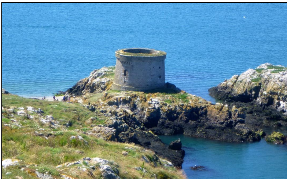
Plate 13 Martello Tower, facing northwest
