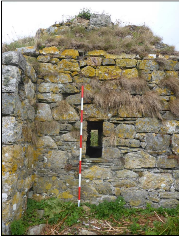
Plate 36 View through both windows of chancel from exterior, facing north
