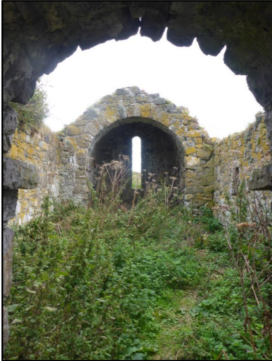
Plate 33 Interior of church: View from east doorway towards chancel
