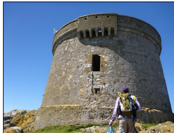
Plate 14 Martello Tower, facing north, showing raised doorway and machiolation
