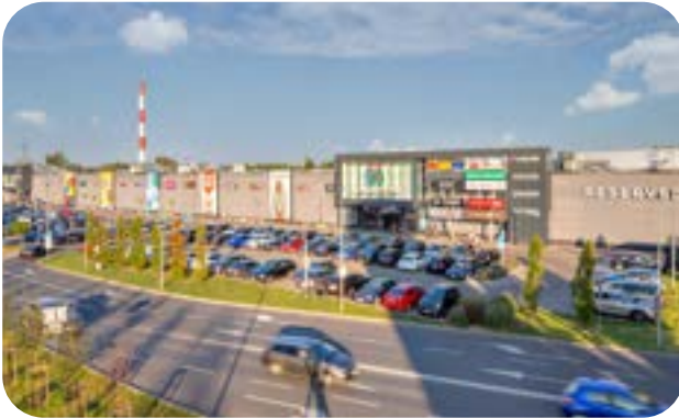
Galeria Wolomin Wolomin
