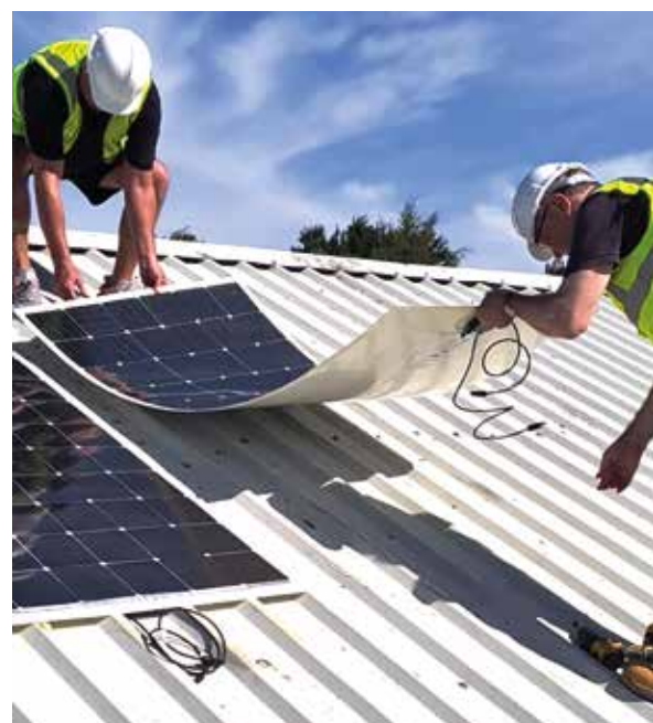
Figure 6 Place flexible solar PV panel on roof.
