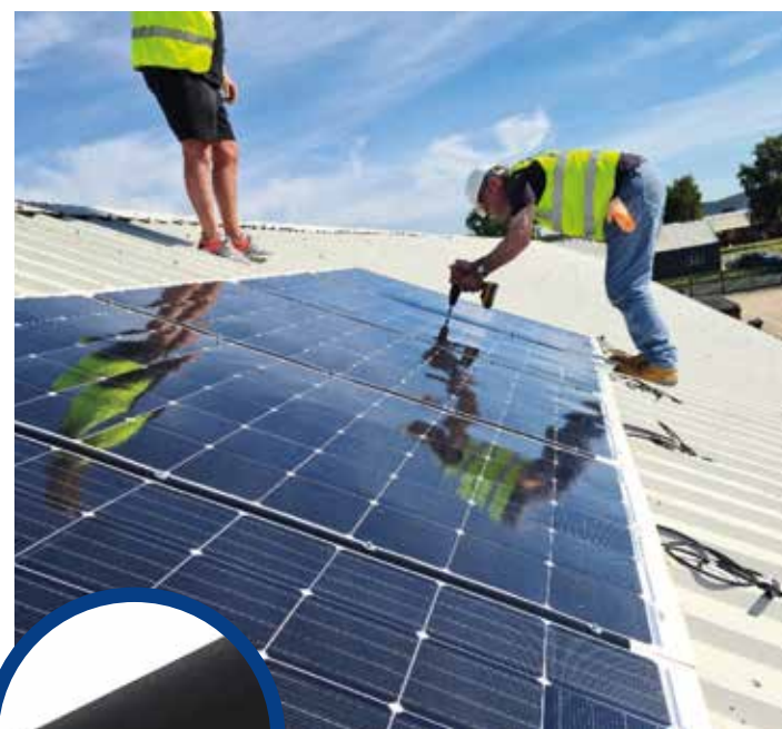
Figure 7 Installing the cover strips between the solar PV panels.
