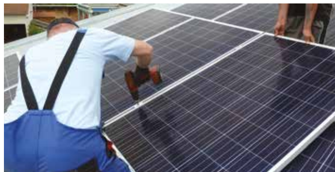
Figure 4 Installing the Mid clamp.
