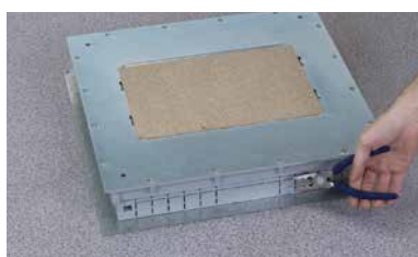
Trim the trunking inputs
