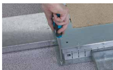
Insert the trunking and bolt to the floor
