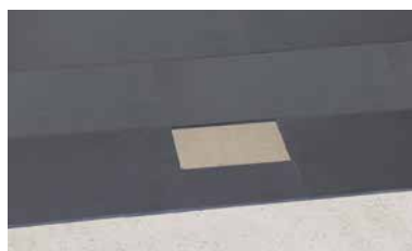
Lay the lining
