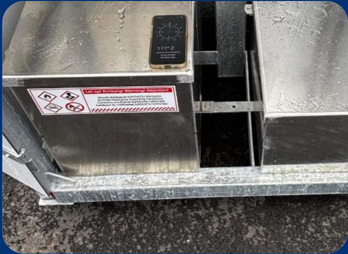
1. Position the tower with the door facing north; a compass app can help with this.
