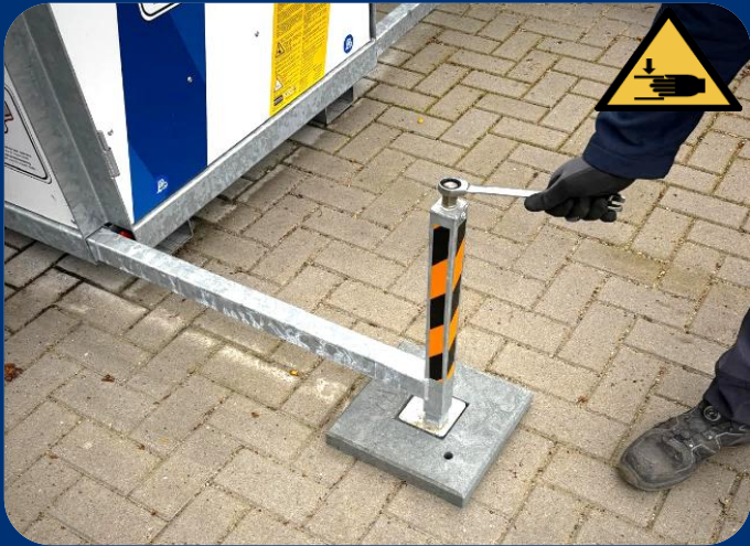
2. Pull the support legs out and place a tile underneath. Use the 19 mm spanner to unscrew the legs. Use this to level the tower.
