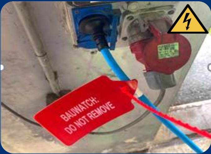
9. Connect the other end to a suitable power outlet, ensuring that the red label is visible so that the cable cannot be easily removed.
