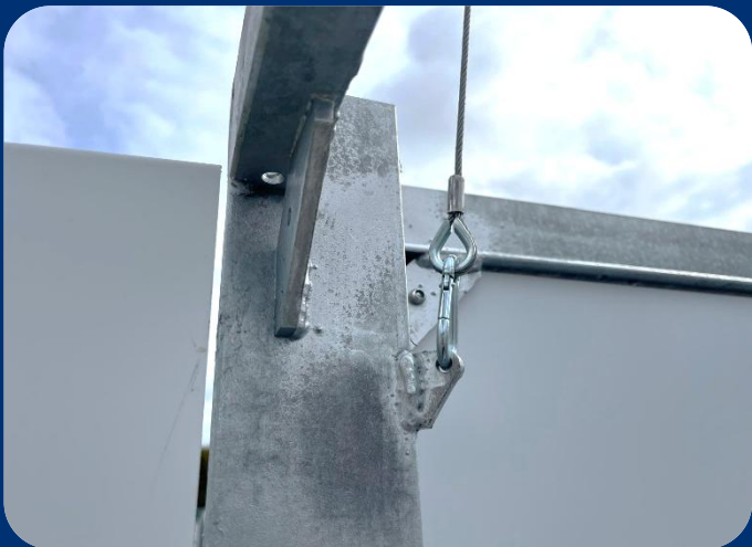
5. Before the mast is fully extended, check the hooks again to ensure they are still secure.
