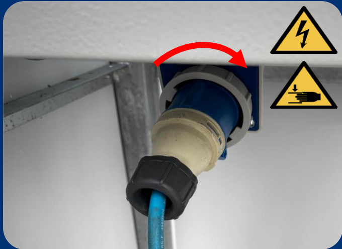
8. Connect the CEE plug to the system cabinet and lock it by turning the retaining ring.
