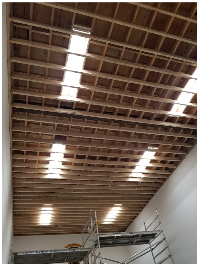
Fig 15.0 – Installation for Ceiling Joists
