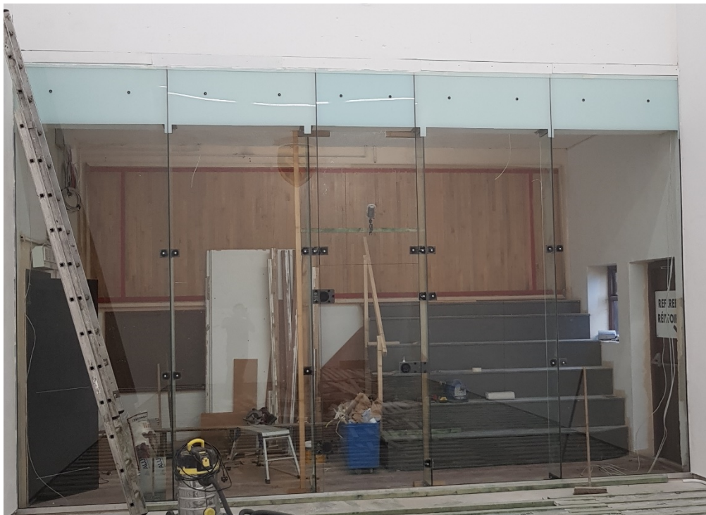
Fig 24.0 – Glass wall Installed
