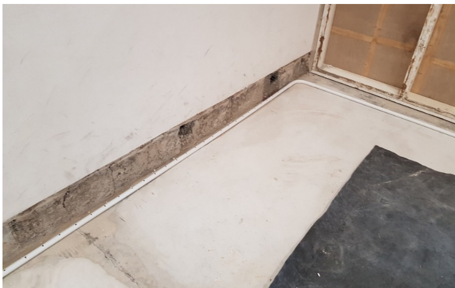
Fig 5.0 – Installation of 25mm Plastic Conduit
