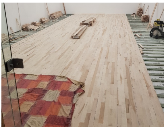
Fig 11.0 Installation of Maple Floor
