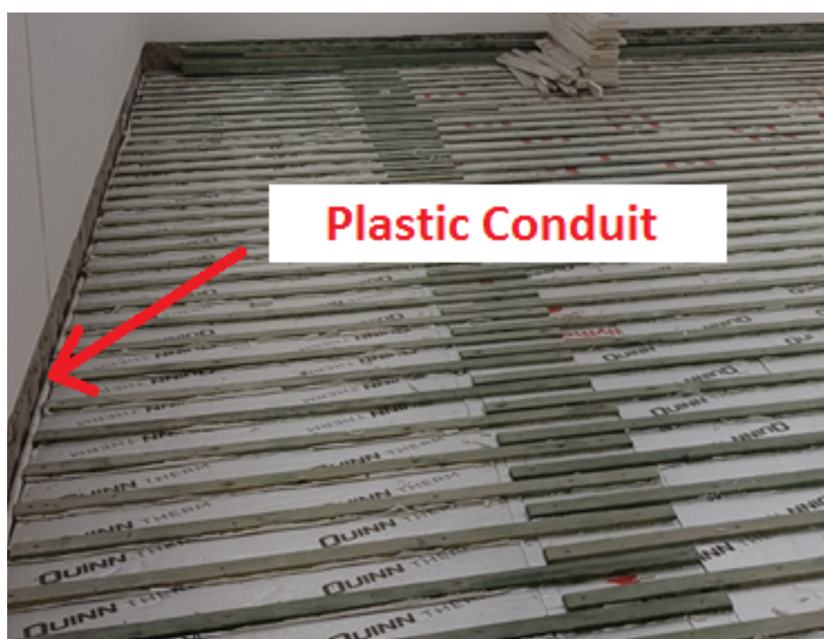
Fig 6.0 – Plastic conduit around perimeter of alley
