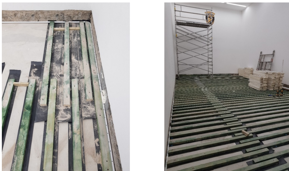
Fig 3.0 and 4.0 – 3"*2" Batten installation
