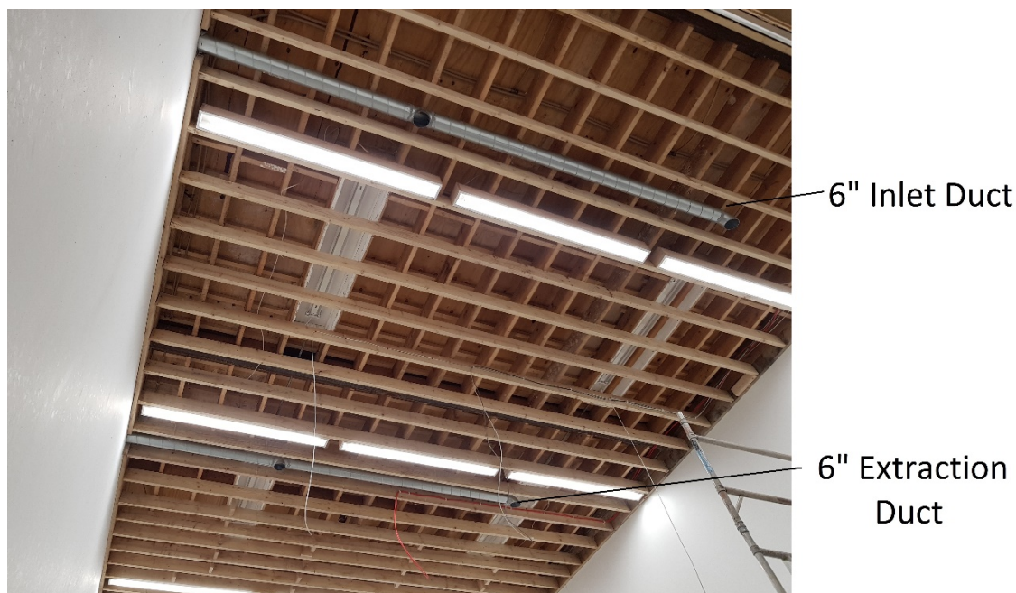
Fig 19.0 – Installation of Spiral Ducting
