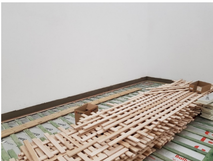
Fig 8.0 – Ventilation of Maple Timber
