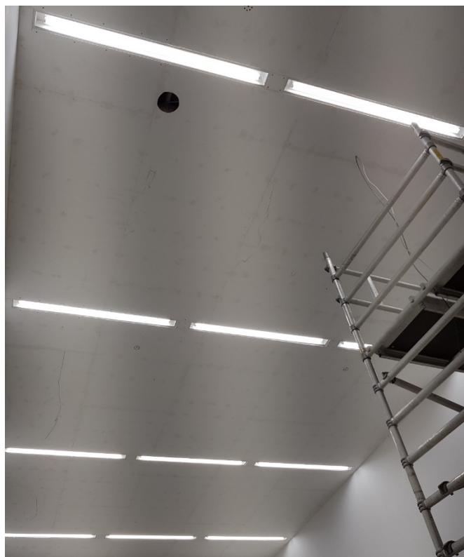
Fig 20.0 Installing Beech Plywood Ceiling
