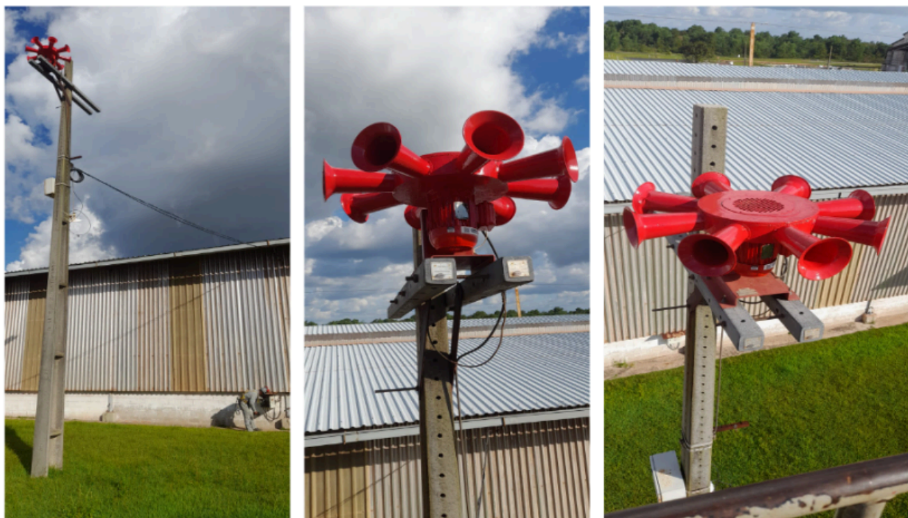
Figura 14-1 – Sirene instalada.
