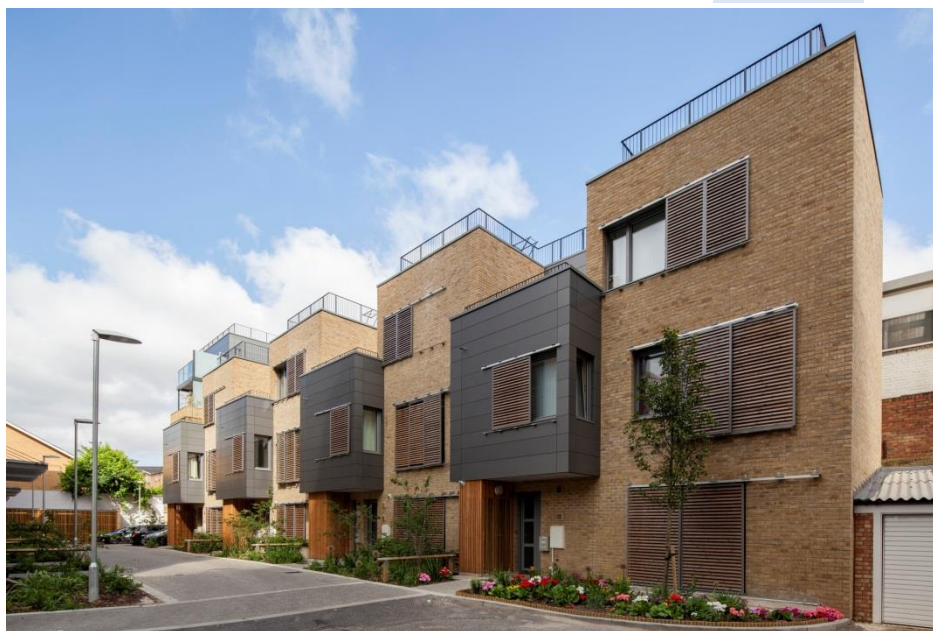
Greenhouses, Sulgrave Gardens, London Insulation & Panels
