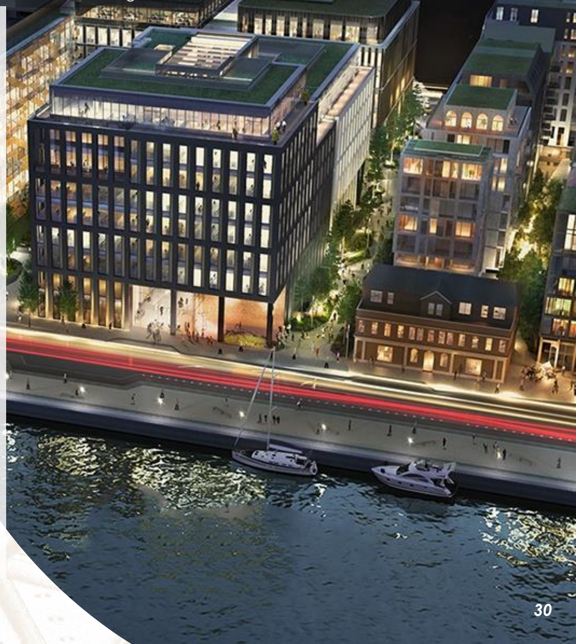
Dublin Landings Dublin, Ireland Data + Flooring
