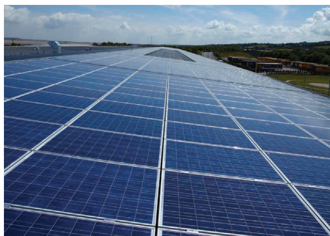
KINGSPAN INSULATED PANELS MANUFACTURING FACILITY, HOLYWELL, UK.
