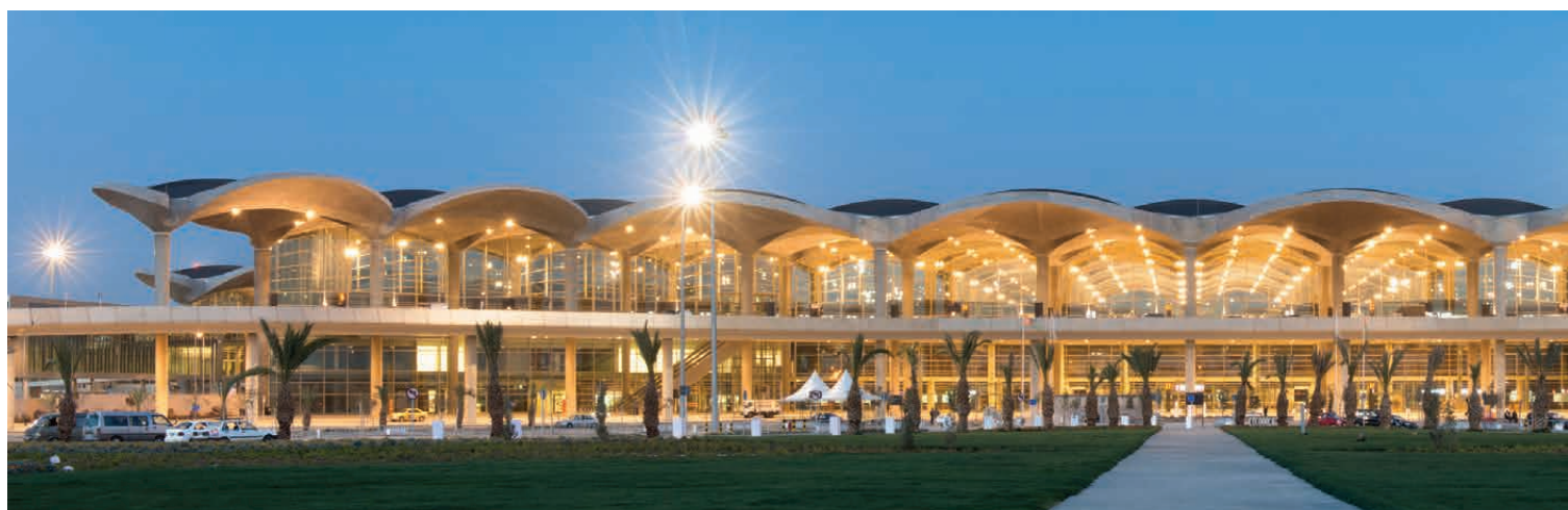
QUEEN ALIA INTERNATIONAL AIRPORT, NEW TERMINAL, JORDAN.
