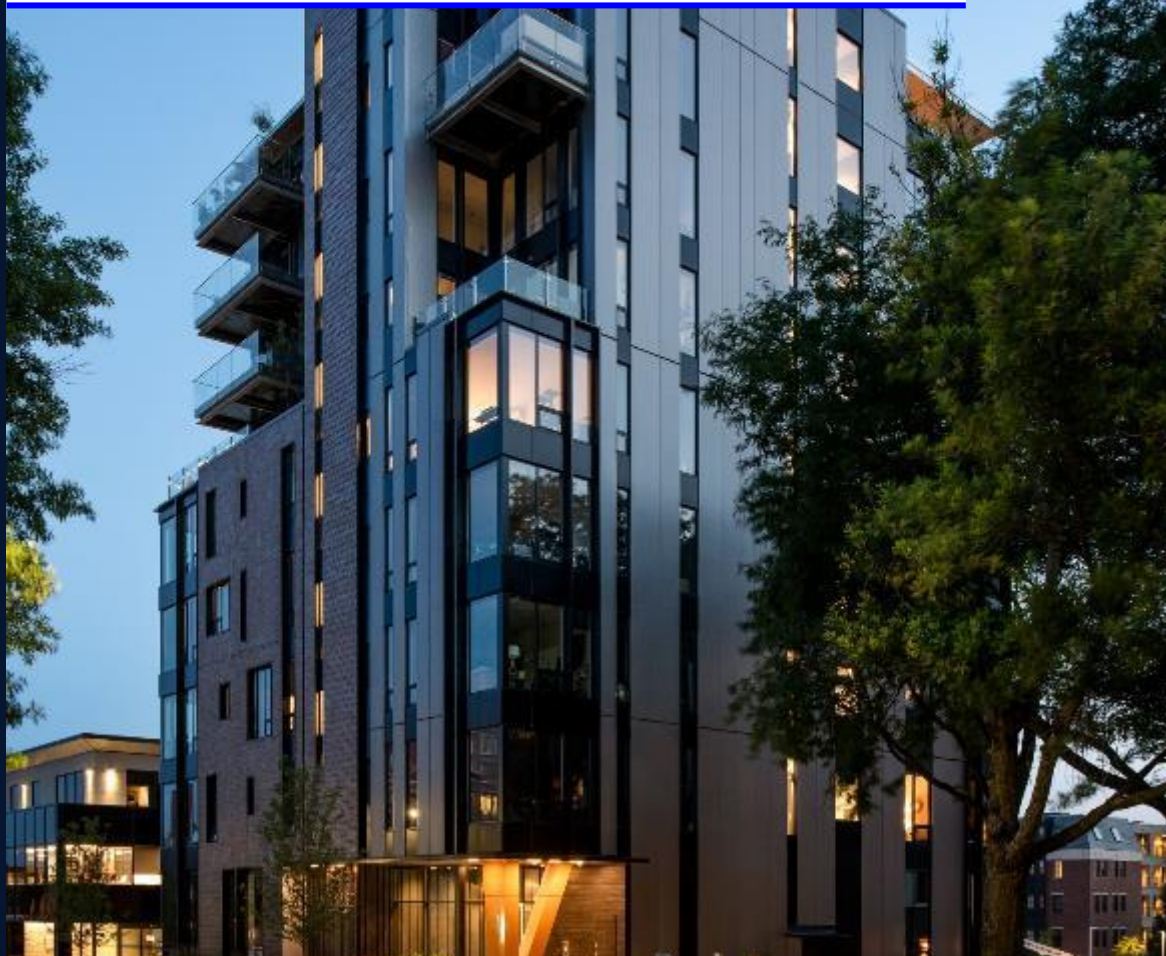
The Nest, Vermont, USA Insulated Panels
