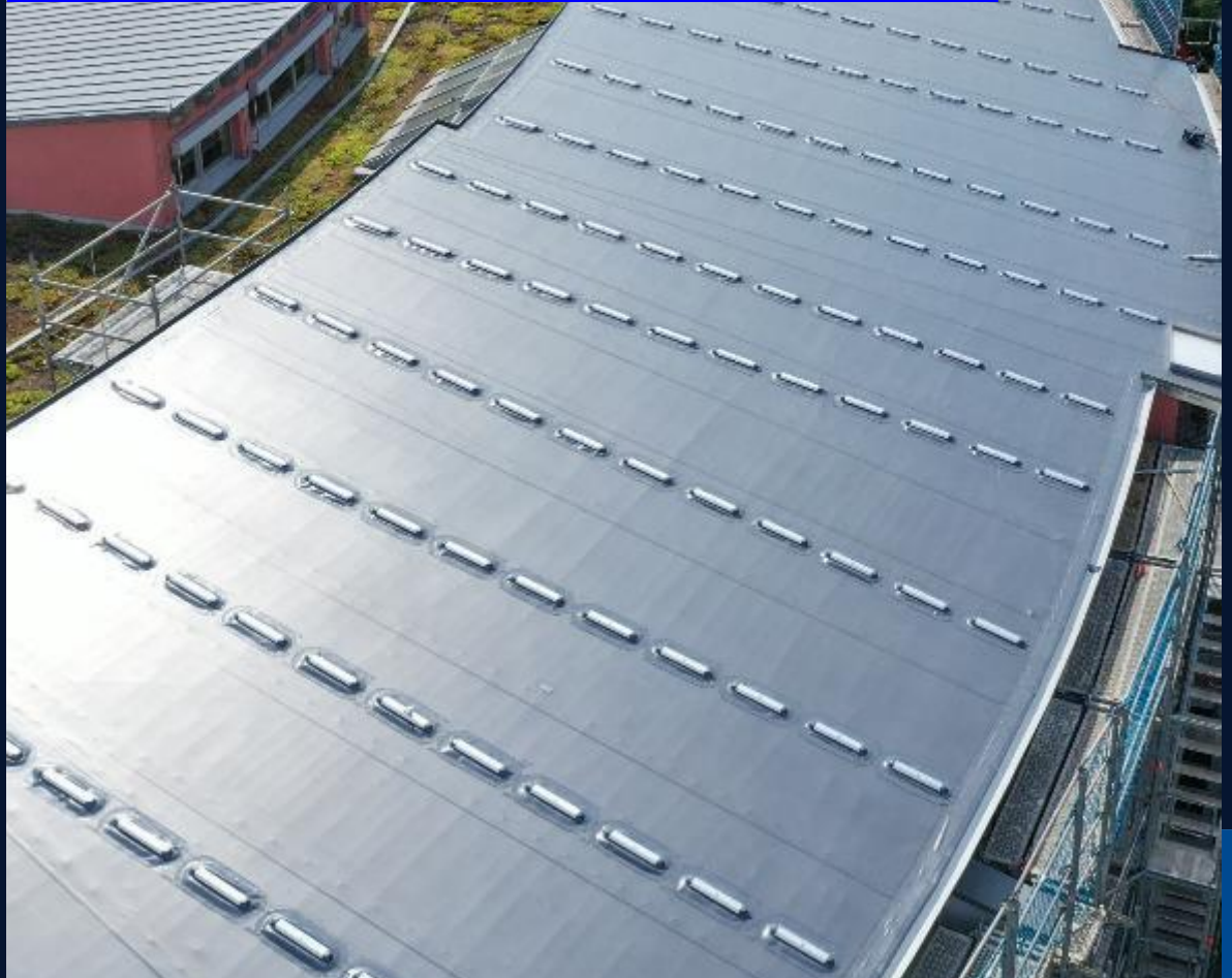
Dietrich Bonhoeffer Gymnasium, Schweich, Germany Roofing + Waterproofing
