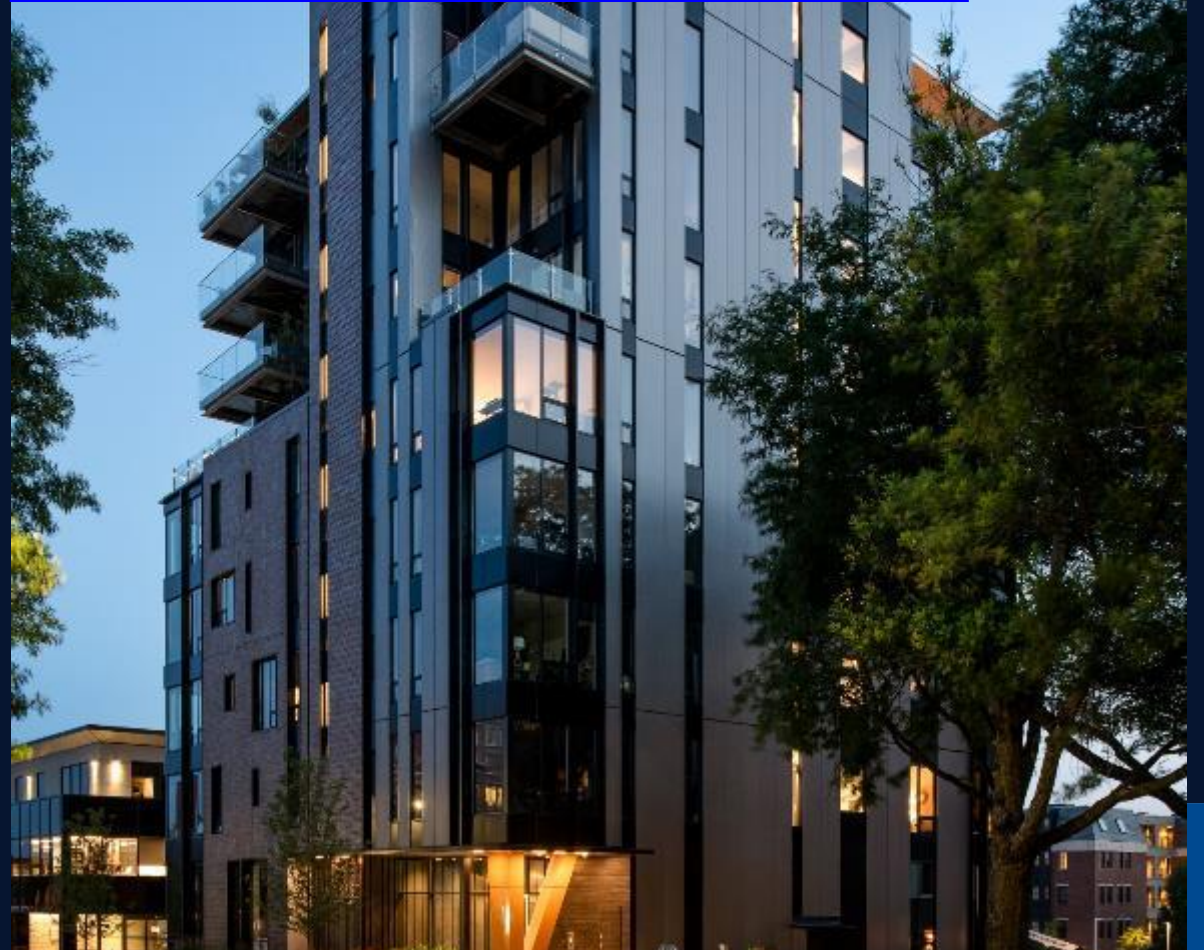
The Nest, Vermont, USA Insulated Building Envelopes
