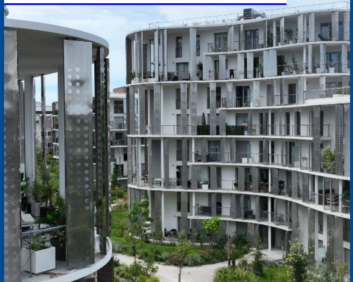
Oxygene, Marseille, France Advanced Building Systems
