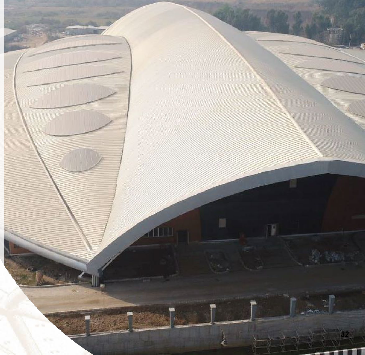
Kartapur Airport India Kingspan Panels
