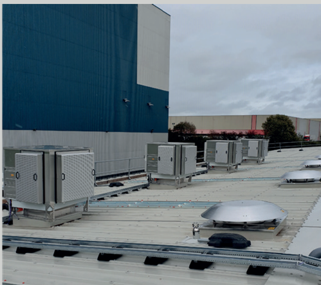
Tornado can be combined with the Colt CoolStream evaporative cooler to provide costeffective air conditioning for industrial and commercial applications
