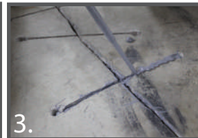
3. Apply epoxy over the Concrete Crack Lock
