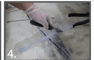
4. Scrape away excess epoxy
