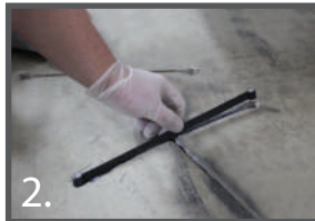
2. Press the Concrete Crack Lock into epoxy
