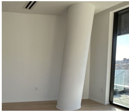
Olympia Dumbo's sail-shaped design presented structural challenges, including the placement of load-bearing, sometimes sloping columns so they didn't interfere with a unit's layout. Photo: Amanda Schiavo/for Commercial Observer
