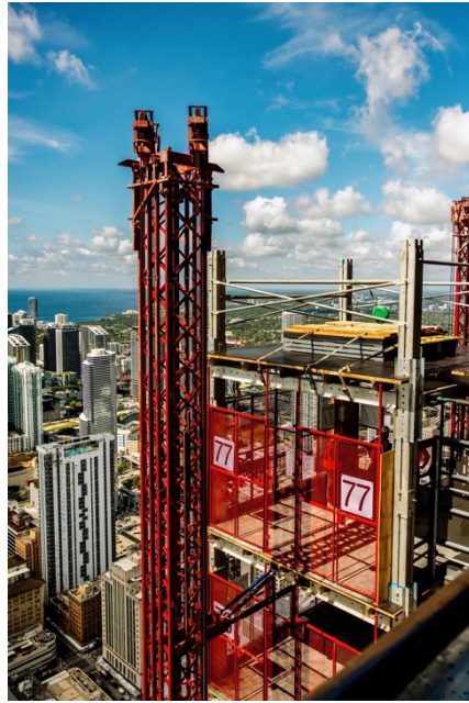
The construction elevator on the Waldorf Astoria currently goes up to the 83rd floor. The skyscraper will reach 100 stories by the end of this year, making it Miami's first skyscraper over 1,000 feet.
