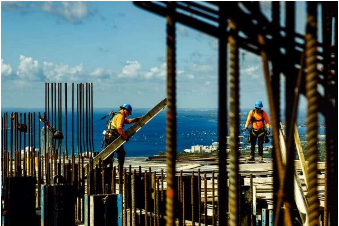
Construction workers on one of the highest levels of the currently under construction Waldorf Astoria Residences in downtown Miami
