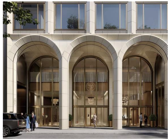
At 520 Fifth Avenue, three grand arches form three separate lobbies.
