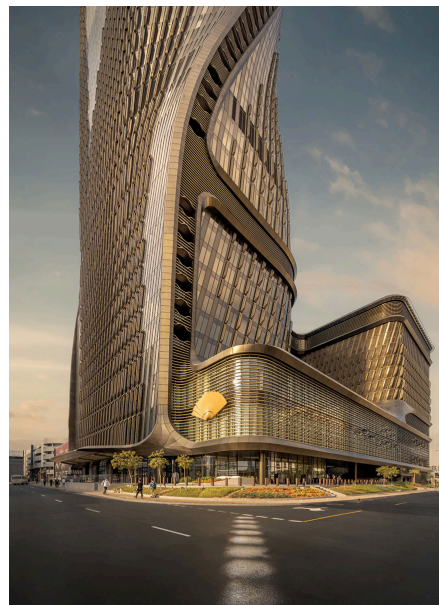
Thousands of fins (1) dot Wasl Tower's facade, which twists from its base (2) toward the sky (top of page). Photos © Ahmad Alnaji
