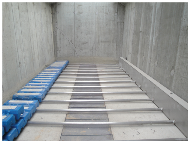
Filter construction/structure
