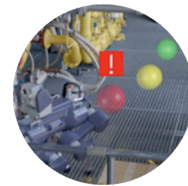
Assessing the presence of gas
