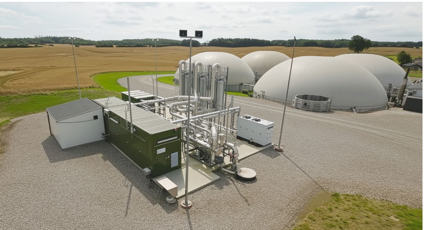
The membrane system in Gråsten, Denmark, produces biomethane that is fed into the natural gas grid
