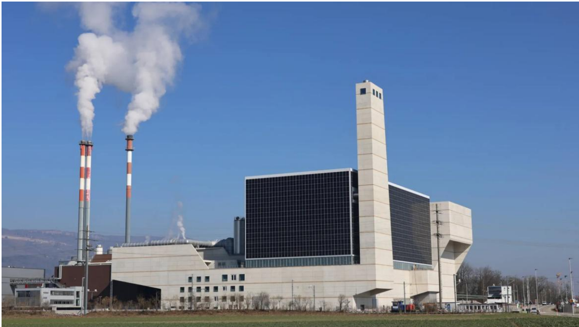
KEBAG_Enova_Emmenspitz.jpg: The new KEBAG Enova Emmenspitz waste-to-energy plant in Zuchwil, Canton Solothurn, Switzerland.
