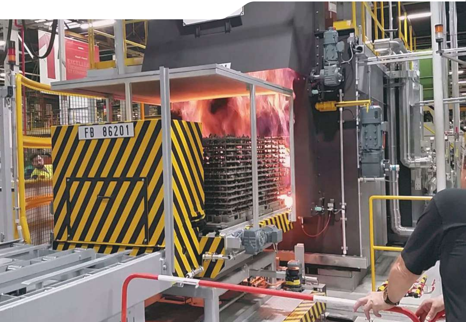
two chamber furnace 1500 kg – 950°C
