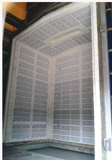
reconstruction of electro heated furnace - after
