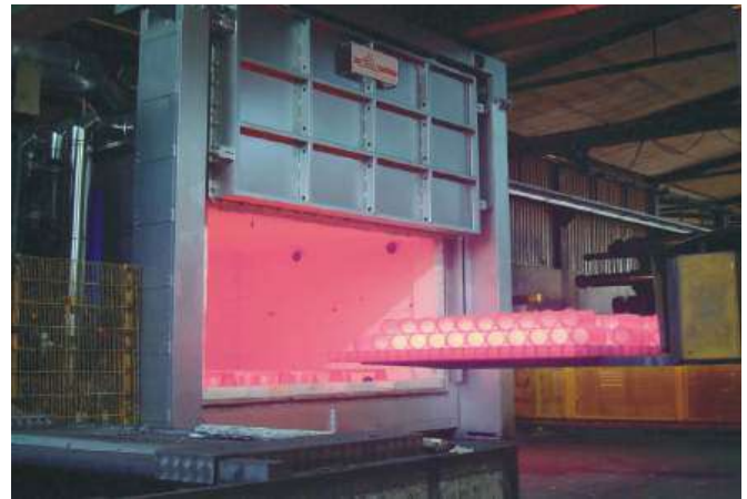
gas heated furnace - 6 m 3 - 1150°C
