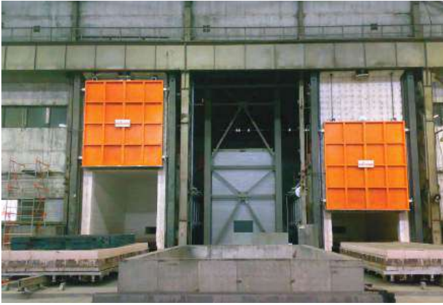
furnace with quench tank
