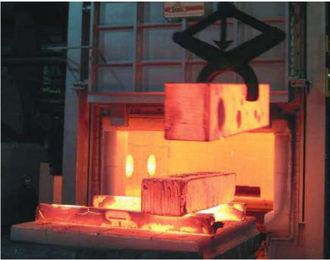
gas heated furnace - 30m 3 - 1300°C
