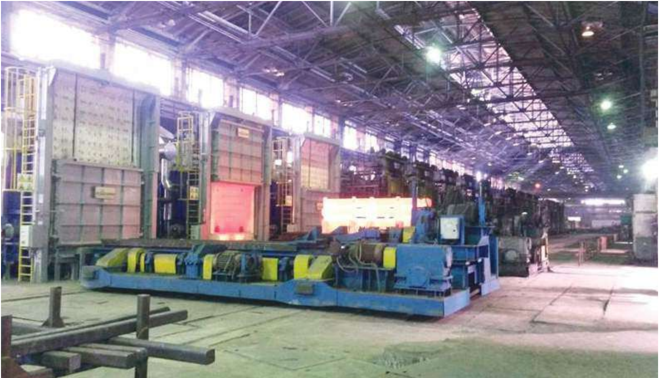
gas heated furnace line with manipulator
