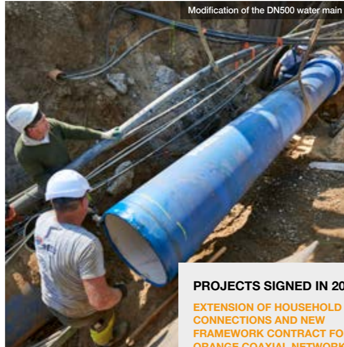
Modification of the DN500 water main
