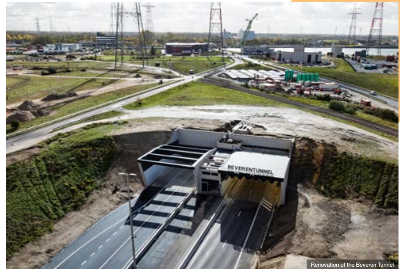
Renovation of the Beveren Tunnel
