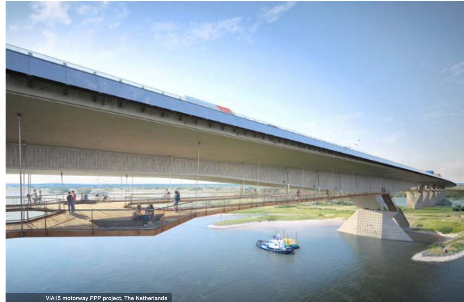
Via15 motorway PPP project, The Netherlands
