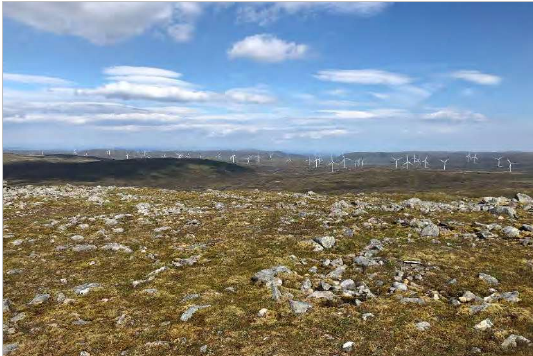
Inset Image A6.3.9: Stronelaig Wind Farm from near to the summit of Geal Charn (926 m AOD) (Assessment Point 4) on the western boundary of the CNP, which despite its presence at close proximity, the vastness of space, scale and height of the surrounding hills of the Monadhliath Mountains and their interior plateau can still be appreciated. (Approx. NGR: 255797, 798527)
