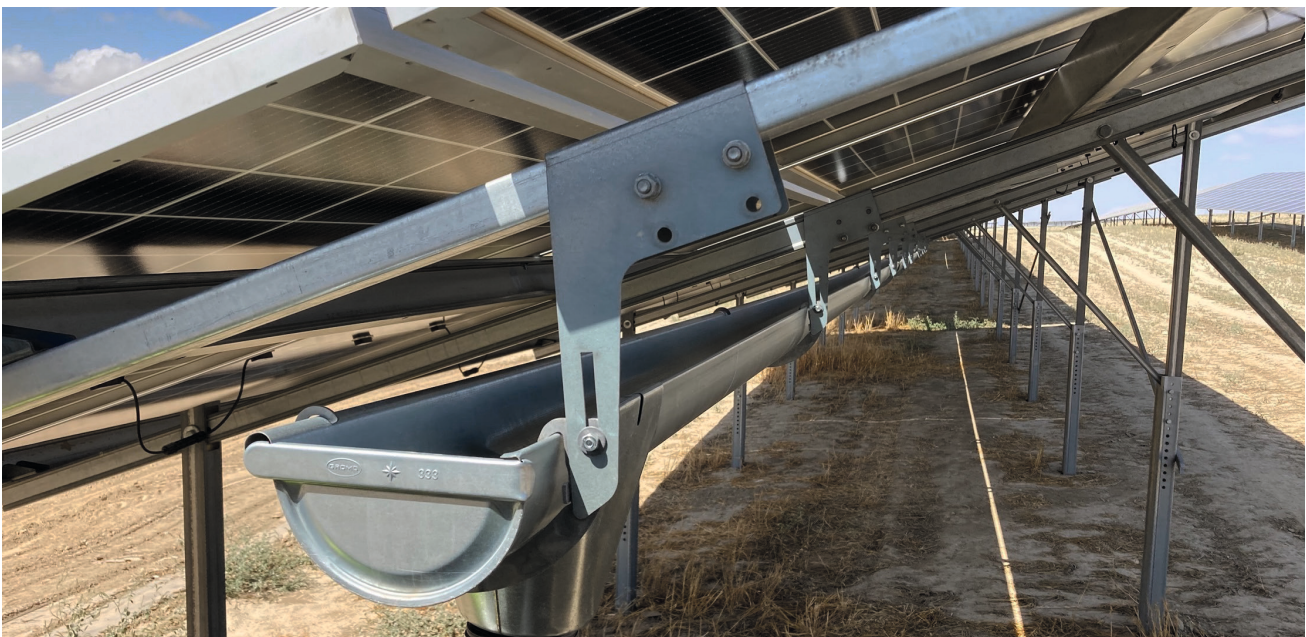
Alhendin Solar Park: Rainwater pipe to collect rainwater and reduce local water stress.
