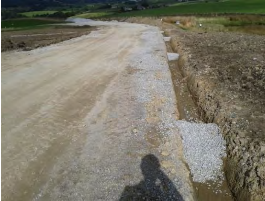
Plate 3.6: Check dam example
