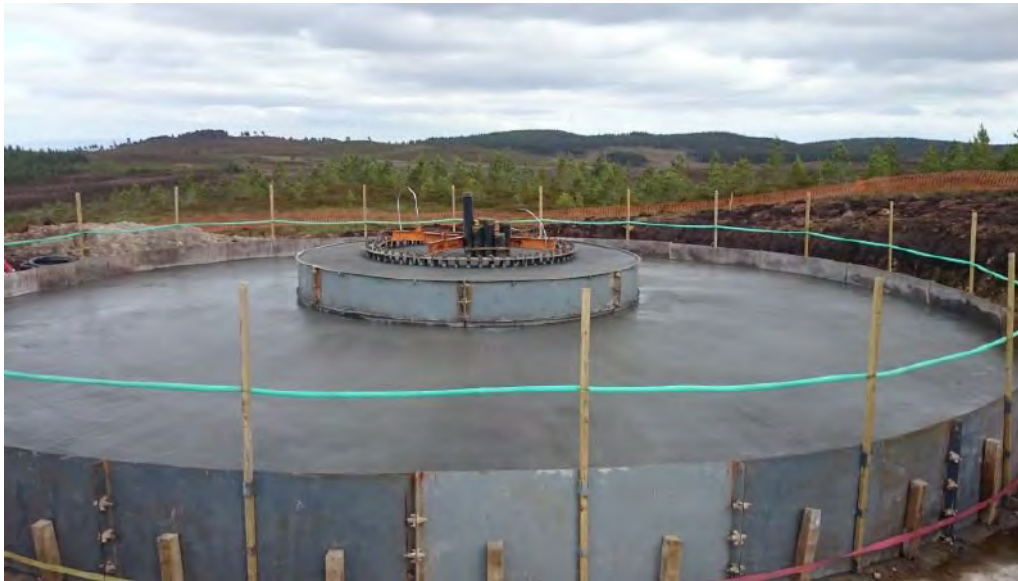
Plate 3.12: Shuttering for concrete foundation (wind turbine base)
