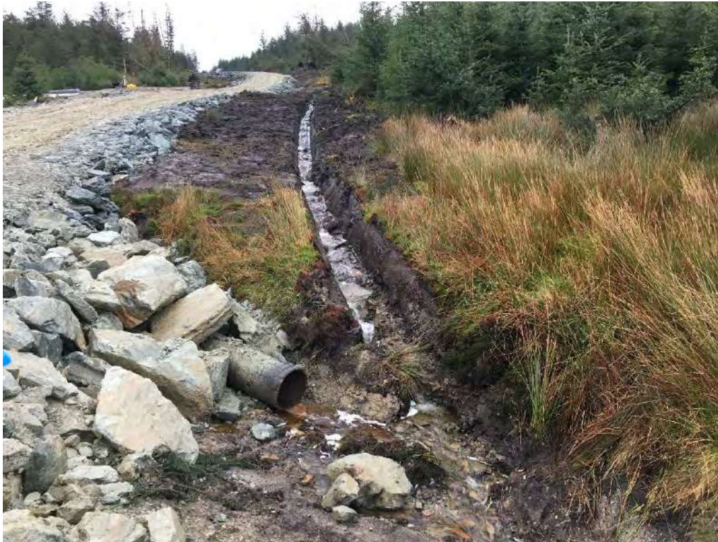
Plate 3.1: Trackside drainage ditch and cross-drainage culvert
