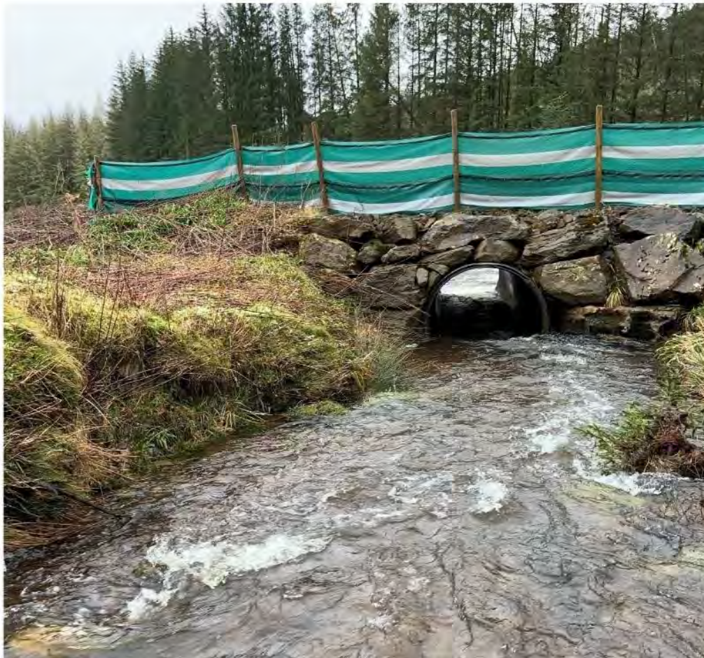
Plate 3.5: Silt fencing at watercourse crossing
