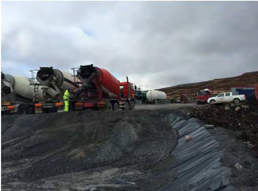
Plate 3.13: Concrete wash-out facility
