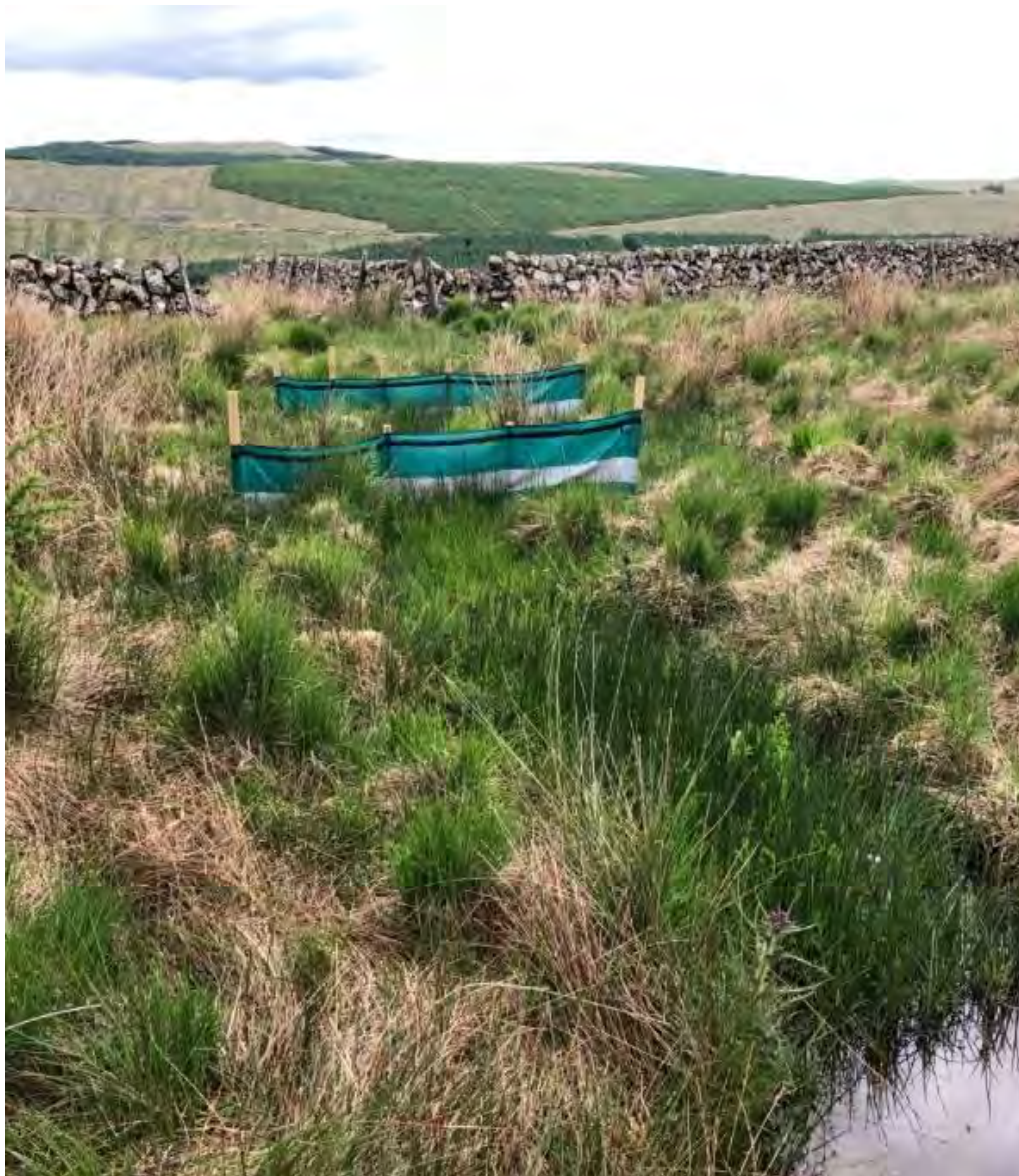
Plate 3.4: Typical silt fencing
