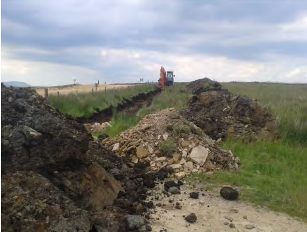
Plate 3.2: Stockpile and drainage ditch (under construction)
