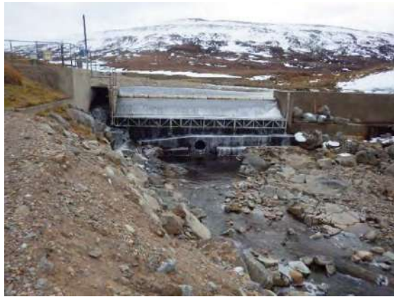
Plate 19 – upstream of CG6 (weir)
